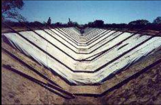
waterproofed coated channels
